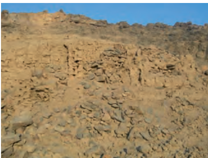
Figure 13. Section of the ancient fortification wall between old Aswan city and Philae temple (built late Middle Kingdom and reused/rebuilt during Graeco-Roman times) showing granite and dolerite stone interior.
